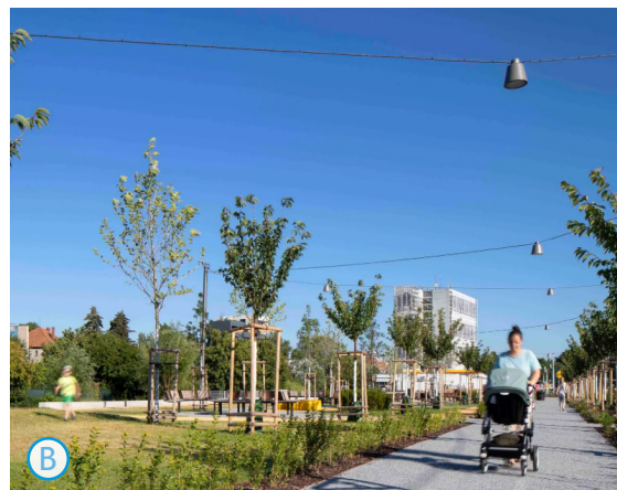
Overhead Lighting at Shared Promenade
