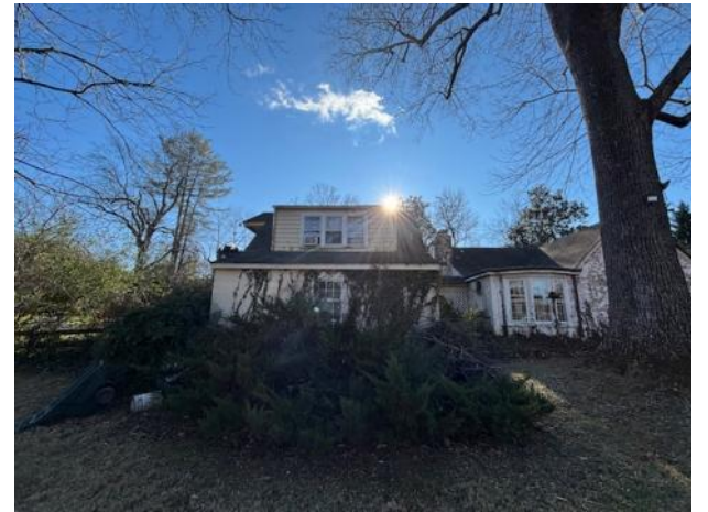
REAR - GARAGE & 1937 PAVILION
