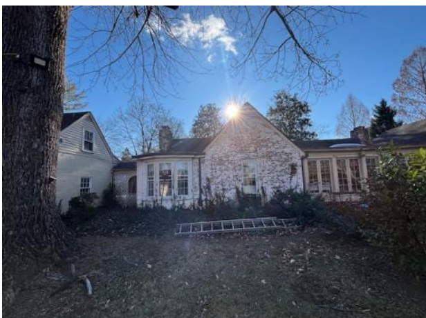
REAR - 1937 PAVILION & ENCLOSED PATIO
